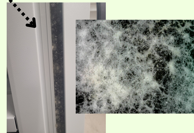
Visible fungal contamination on the compactor sheaths
